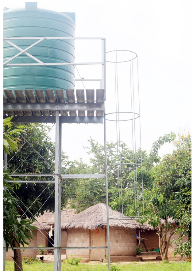
Solar-powered water system and quail houses at Umodzi (Photo – Vincent Eliya)
